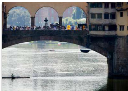
Reconstruction of the facades of the jewelers located on the Ponte Vecchio in Florence and cleaning of Ponte Vecchio
