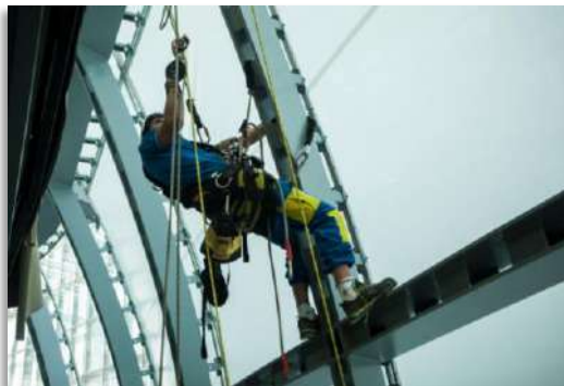
Coating and supply and installation of life lines
