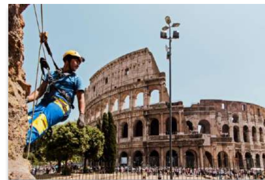
Cleaning and restoration with special mortars of the walls of the Temple of Romulus
